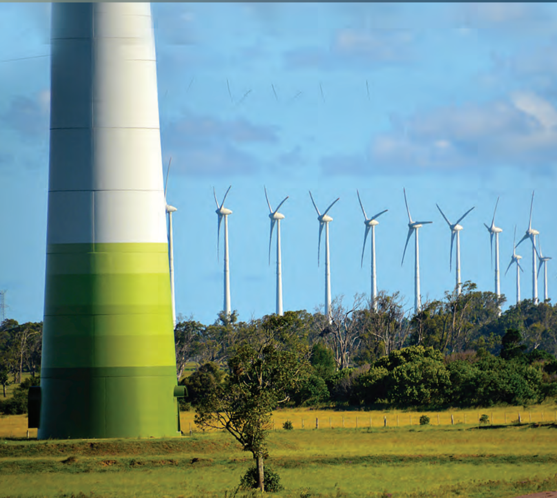
Concrete towers at the Osório Wind Farm
