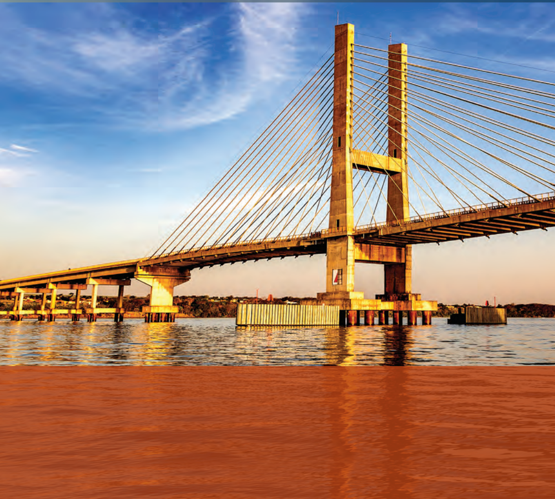
Cable-stayed bridge over Rio Paraná, between São Paulo and Mato Grosso do Sul
