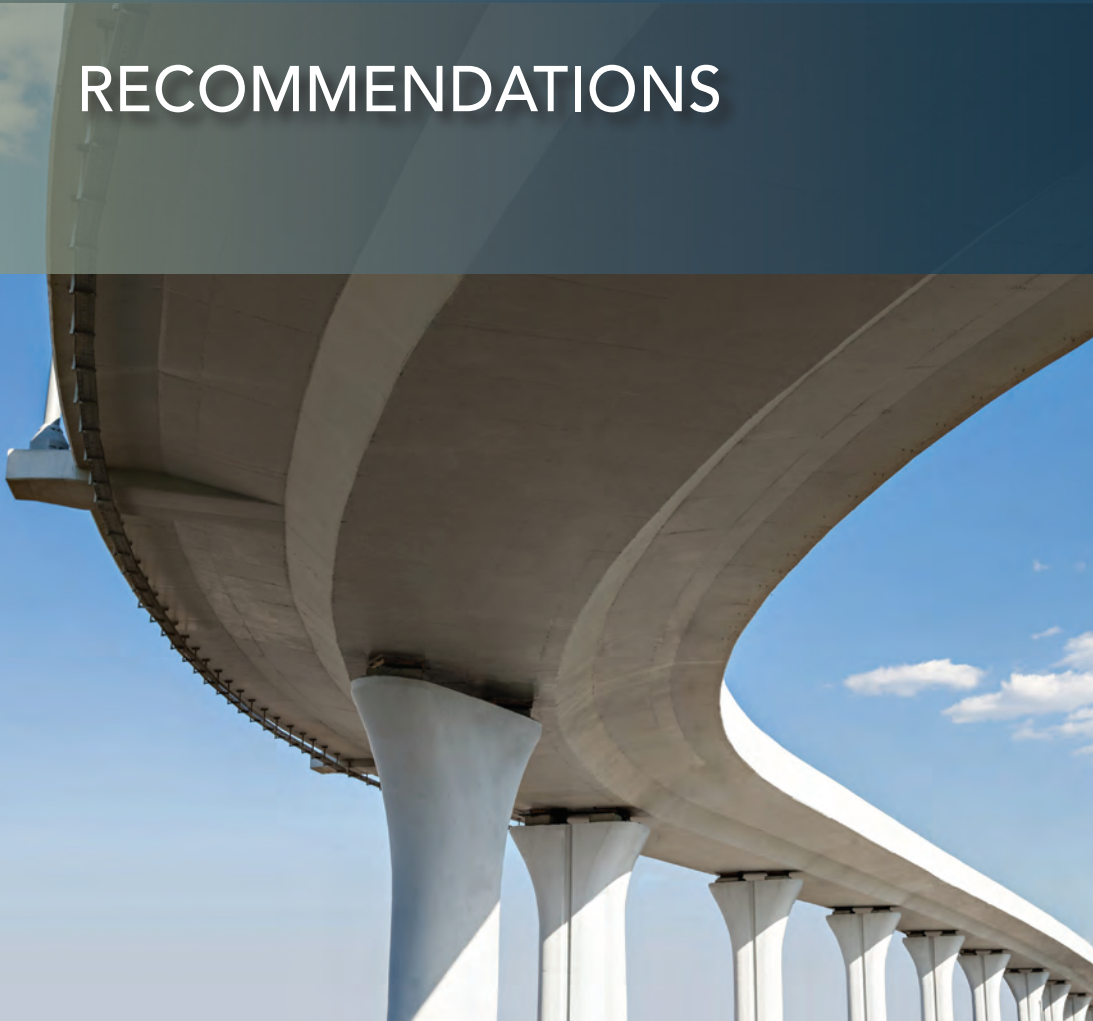
Overpass built in concrete
