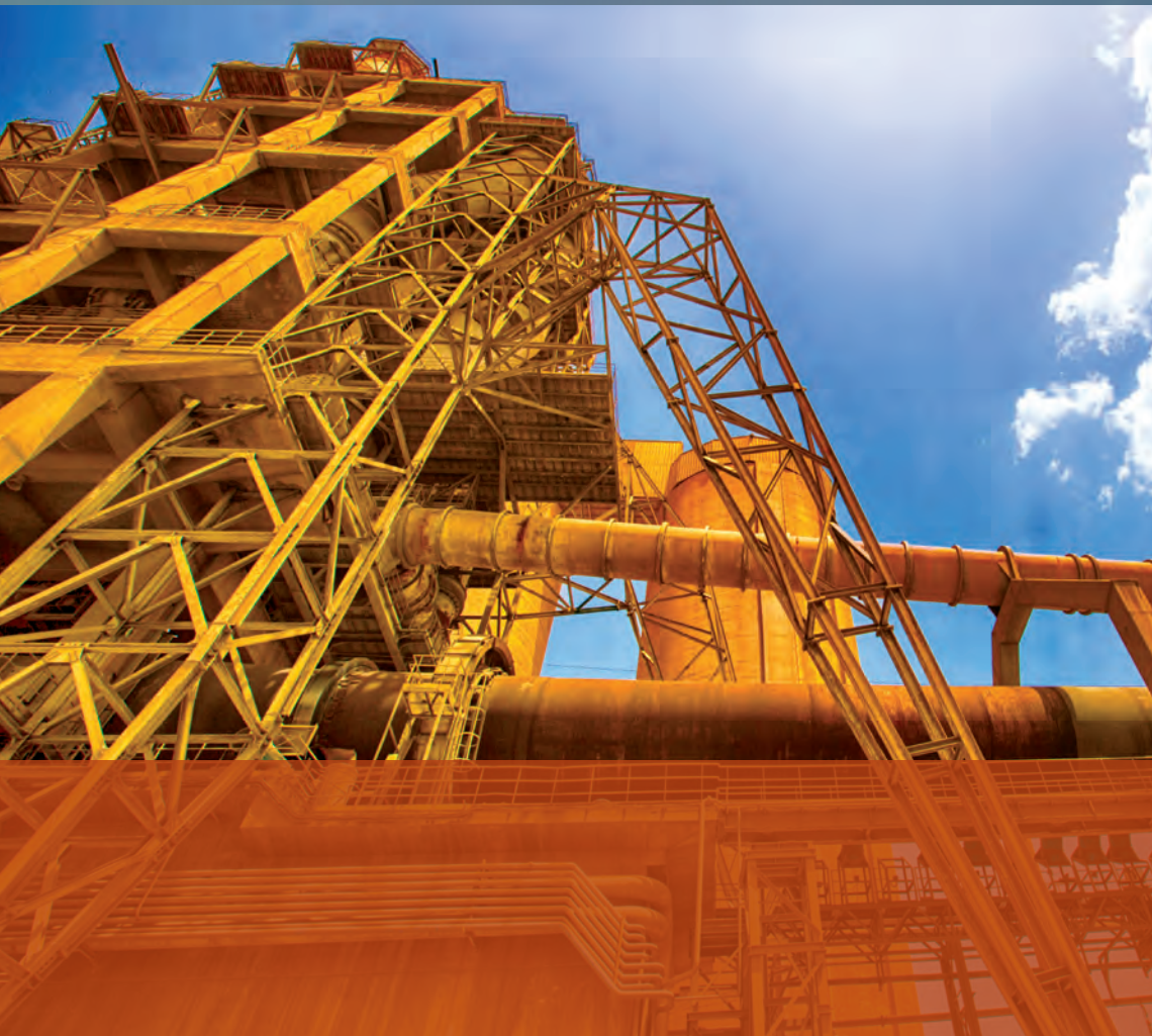
View of the preheaters and precalciner tower
