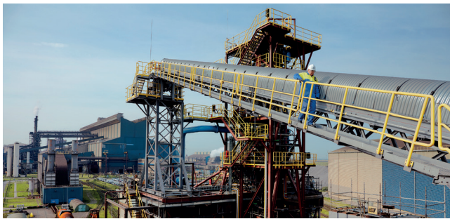
Hlsarna®-Pilotanlage, Tata Steel in IJmuiden
