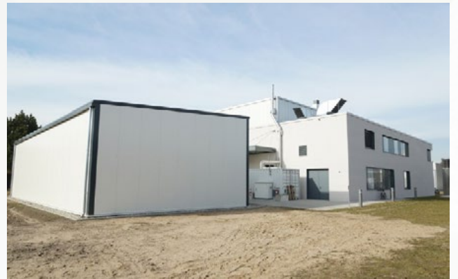
Picture: Pilot plant | Celitement
